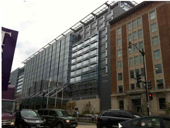
Marriot Marquis & Convention Hall 전경
